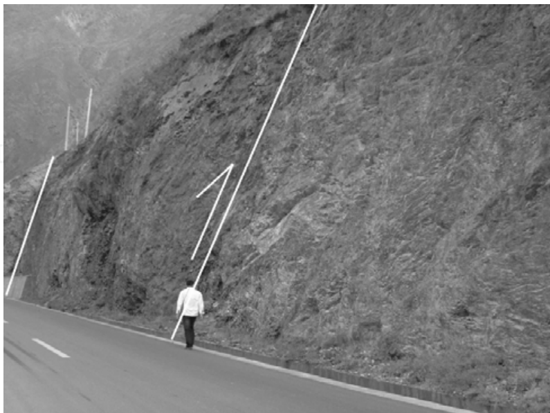
Fig. 7. Western boundary fracture of the Minshan block, (camera facing south) The fault zone is composed of cataclastic rock and fault gouge Carbonization is obvious, fault zone width 20-30m
