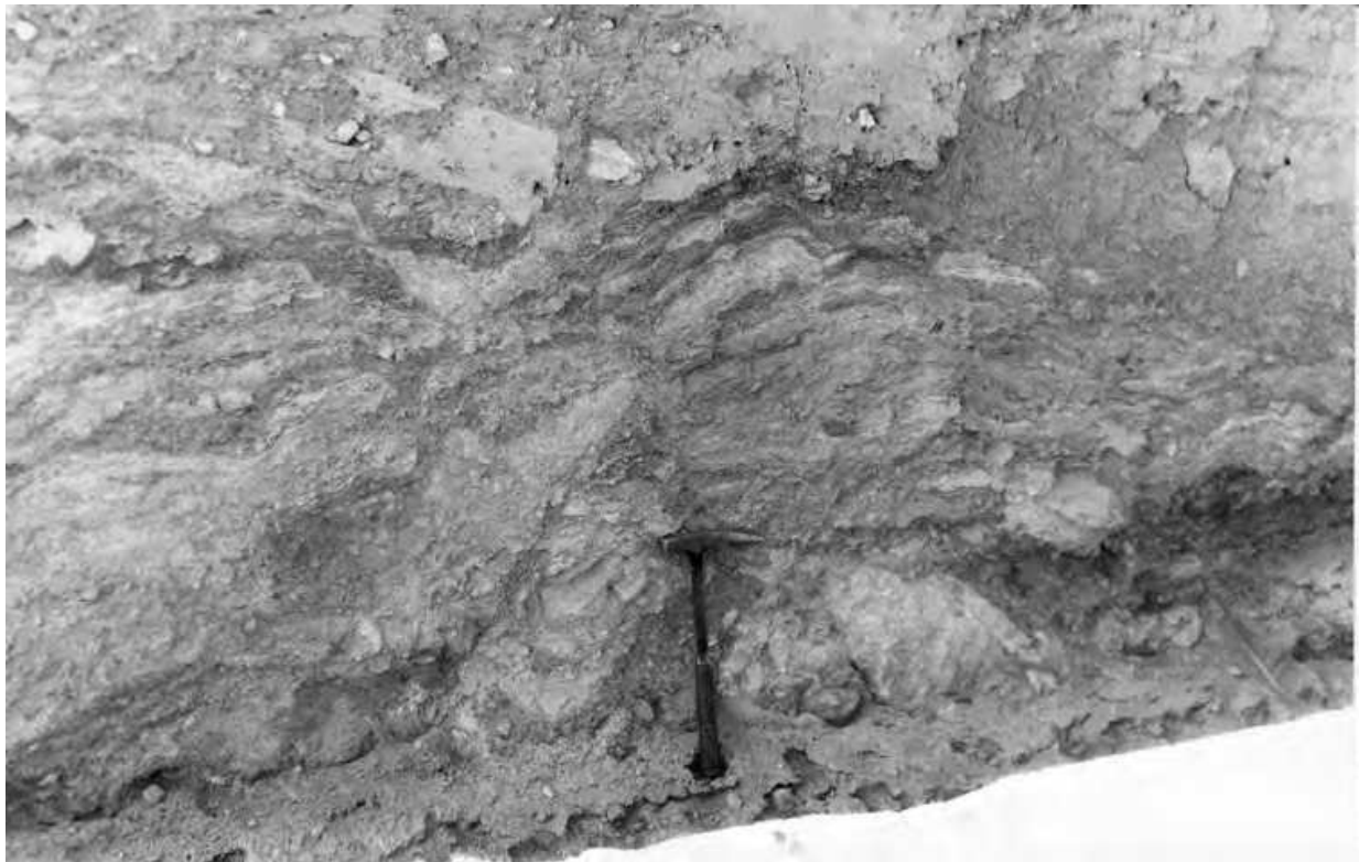
Fig. 22. c. A structure of the Talas-Fergana Fault zone in the Aktaybulak-Korumtokay interfluves. Fault gouge, filled the fault zone, is overlaid by folded alluvial deposits, in which fragments blue clays laying below are found.
