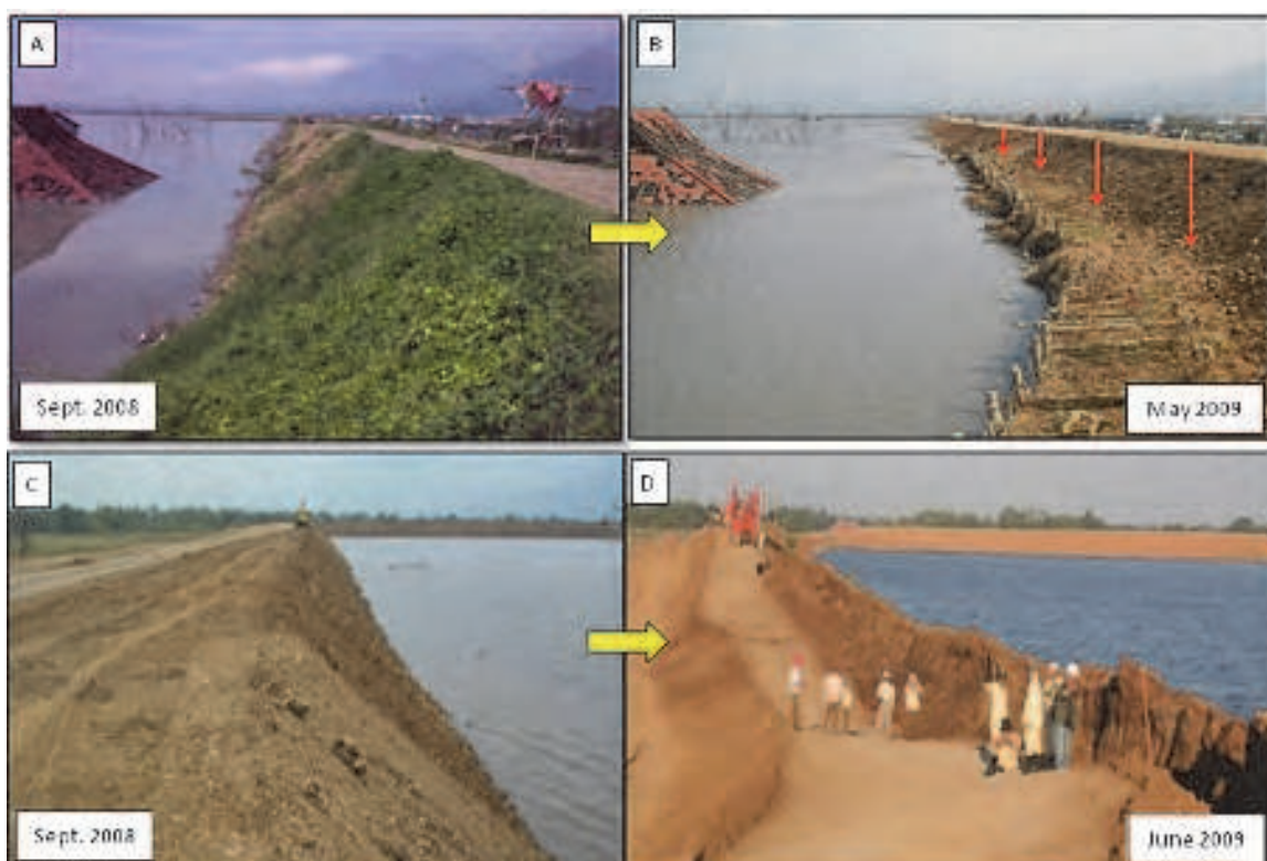
Fig. 28. (A)&(B). Photos before and after the collapse of levees west of the main vent. The levee has decreased in height by approximately 1 meter along a 150 m interval. (C)&(D). Photos before and after the collapse of the levee north of the main vent. The levee has decreased in height by 1.5 m along a 200 m interval.
