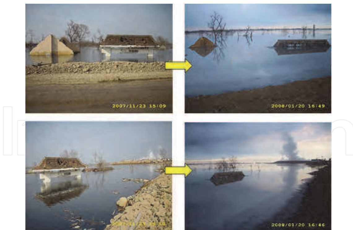
Fig. 27. Dramatical sinking of a village gate of Siring Timur, located to the west of the main vent. The gate and the rubble was half buried but still visible in the 23 November 2007 photograph. Two months later just a part of the tile roof and walls remain visible on 20 January 2008.
