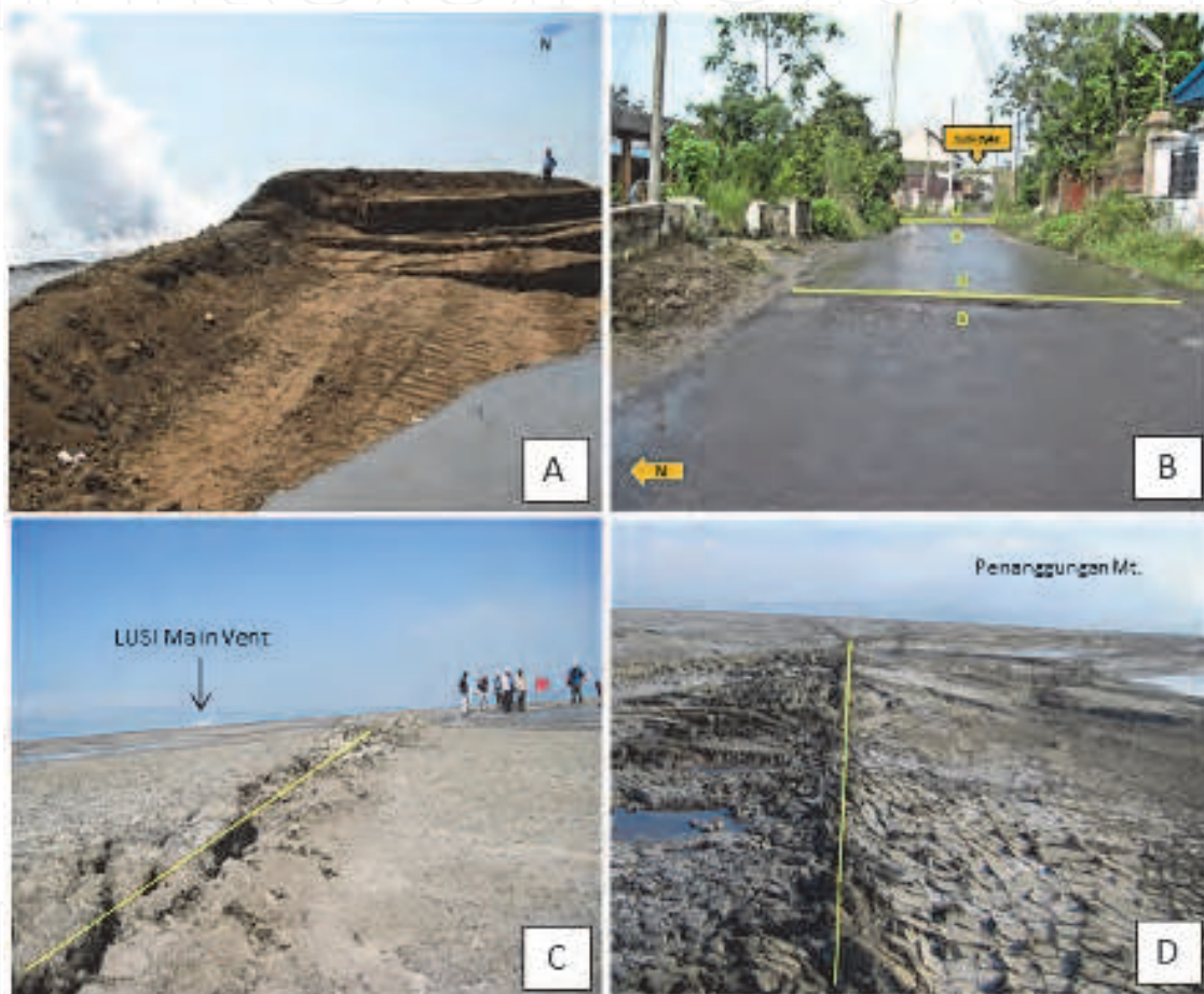
Fig. 21. (A). On June 2, 2008 the dyke on the East side of the main vent broke with an orientation NE-SW. Then on June 8, 2008 the 40 m long dyke collapsed as deep as 6 meters. (B). Fractures on the West Siring village west of the main vent showed an orientation trending North - South. (C)&(D) an active fault is located west of the main vent and trends North - South.
