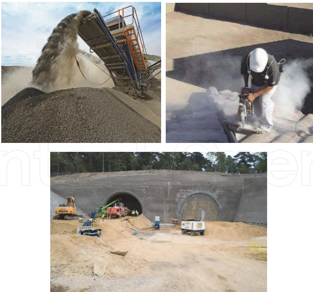
Fig. 1. Job processes that generate and disperse respirable silica dusts into the air
