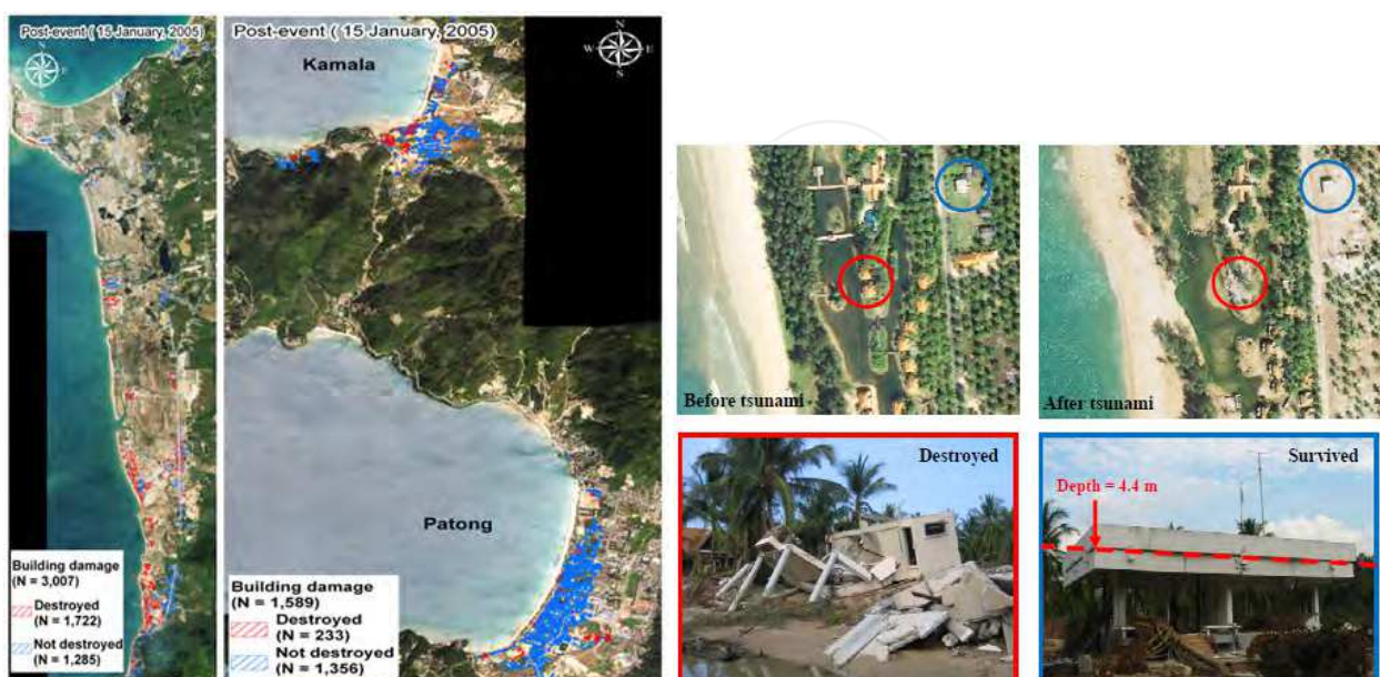
Fig. 10. Visual damage inspection results in Phang Nga and Phuket, Thailand
