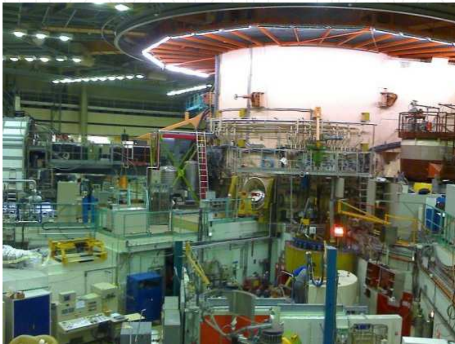
Fig. 13. Inside the reactor hall at ILL in Grenoble (France).
