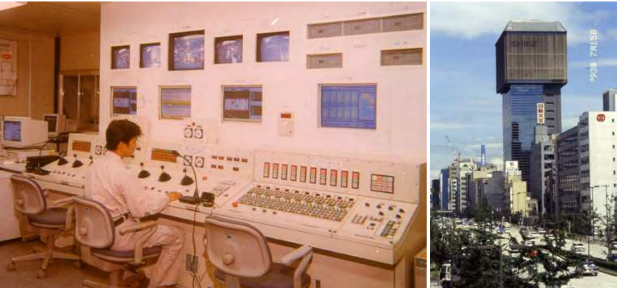
Fig. 16. Control Center of Shimizu’s automated construction system for highly automatic erection of high-rise buildings, Japan, Shimizu Corporation
