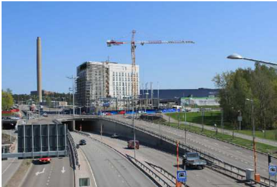
Fig. 11. Photo of the Skanska building partly ready.
