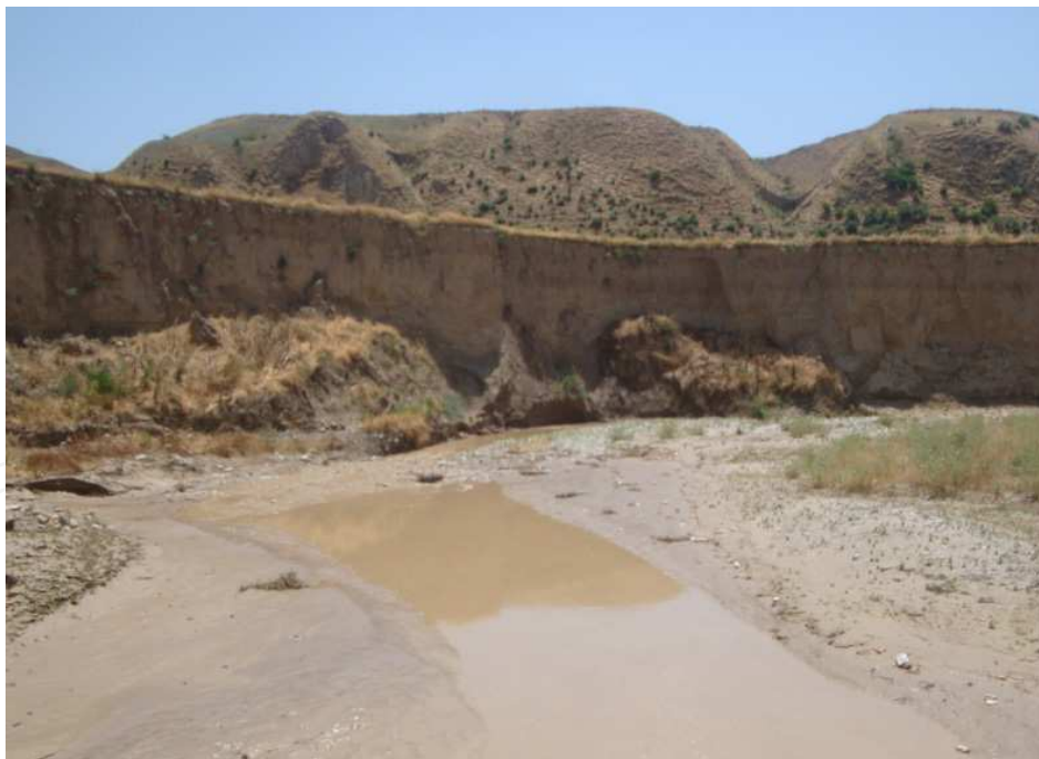
Picture 12. Bank erosion (adjacent to Haji Beik Village)
