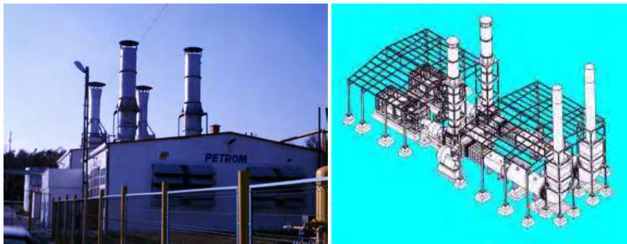
Fig. 1. 2xST 18 Cogenerative Power Plant view (left) and gear placement (right)
