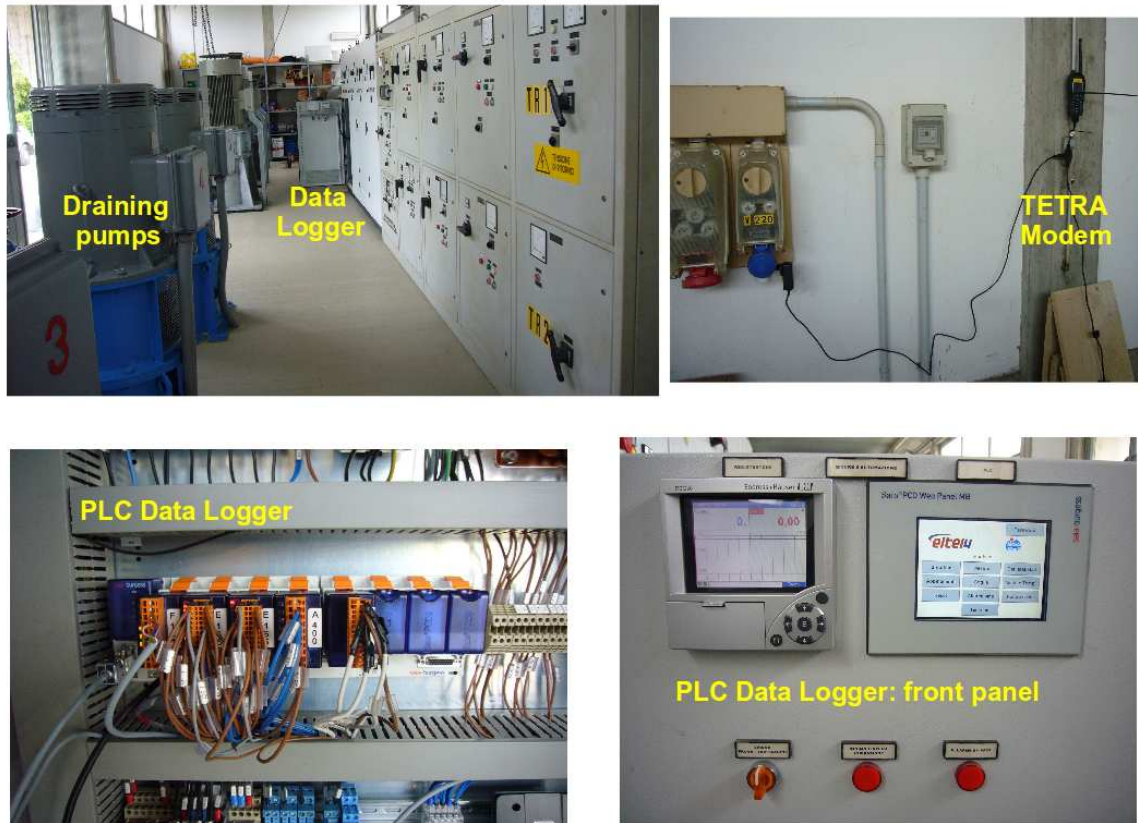
Fig. 9. Draining pump located at “Mordano” city.
