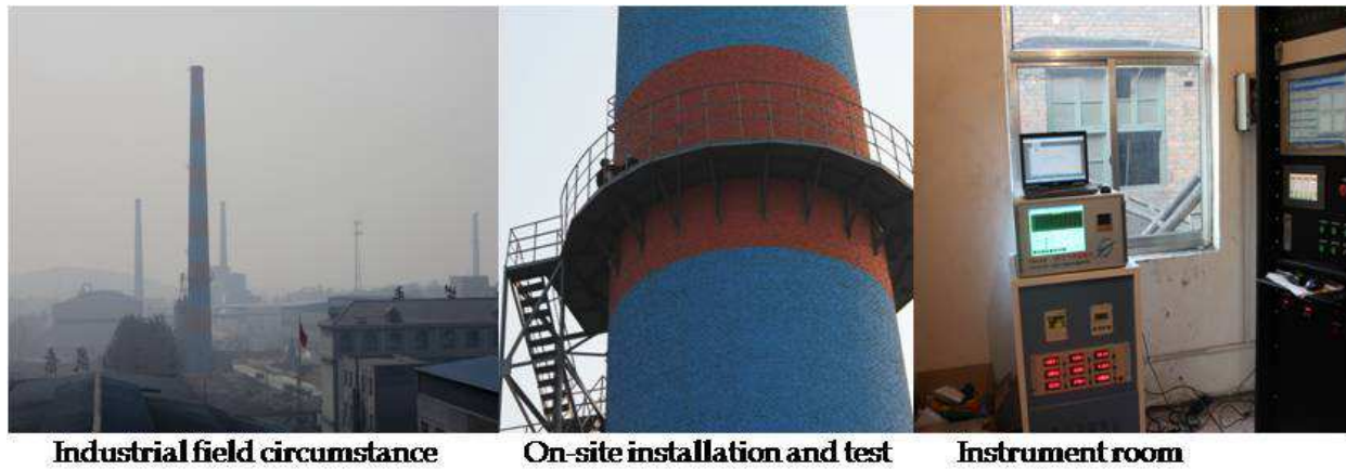
Fig. 16. One of the testing circumstances for in situ on-line monitoring of industrial emissions.
