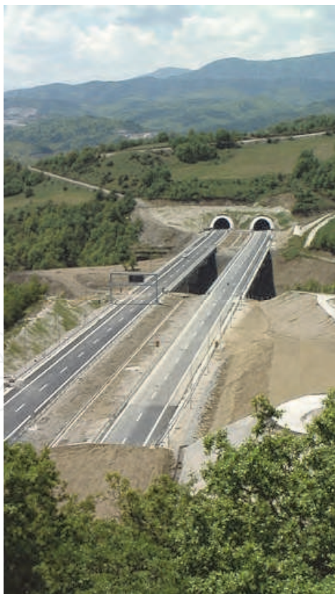
Photo 4. Partial view of the mitigated Egnatia Highway
