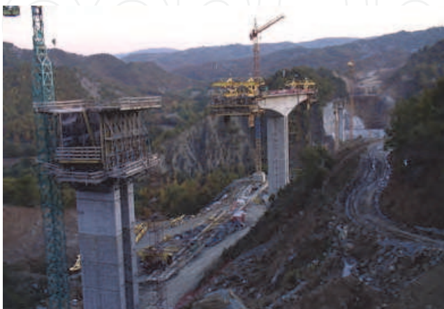
Photo 1., 2. and 3. Construction of the Egnatia highway
