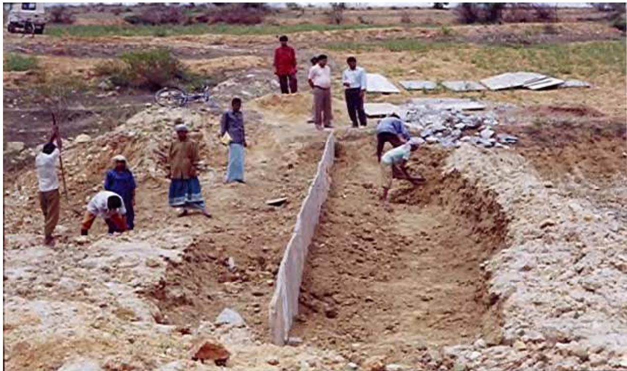
Fig. 17. Providing sub-surface drainage to manage soil salinity/alkalinity
