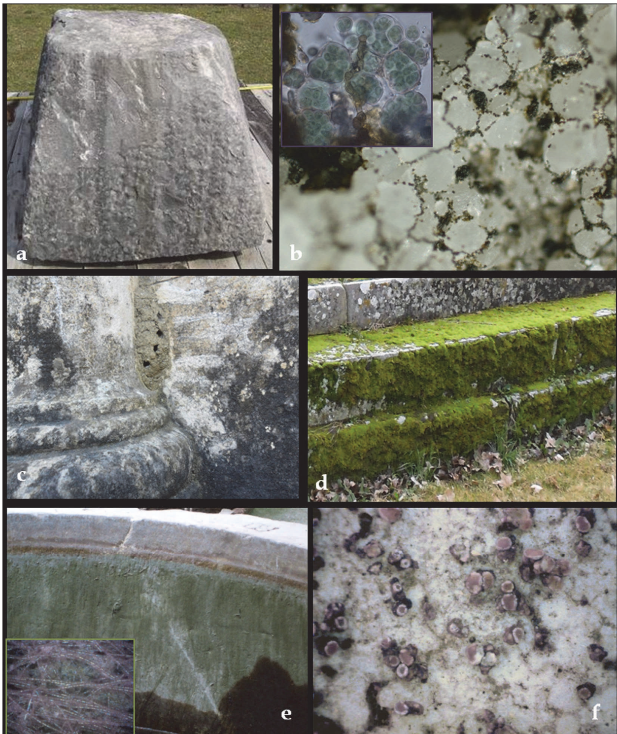
Fig. 7. Different patterns of biological growths found on monumental stones: (a) homogenous black crust with a detail (b) of interganular development of threadlike microcolonies containing cyanobacteria and black fungi, as revealed by microscopic insight, Carrara Marble Museum, Italy; (c) heterogenous lichenic black crust with a wasp nest on a limestone tomb, Trespiano monumental cemetery; (d) bryophyte extended carpets, Fiesole archeological site, Italy; (e) fibrous microbial mat with a filamentous diatom ( Melosira sp.) as a dominant species, Lindaraja Fountain from Alhambra complex, Granada (Spain); (f) micropits containing the apotheci of an endolithic lichen, Trespiano monumental cemetery
