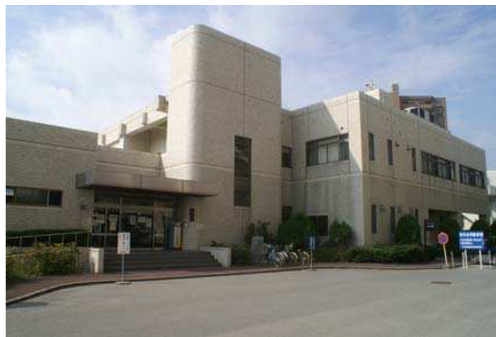
Fig. 13. Yamaguchi University library building
