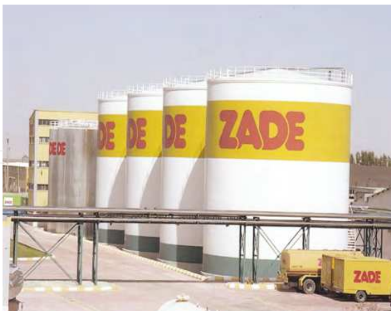
Fig. 5. Crude Vegetable Oil Silos
