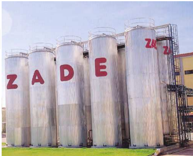
Fig. 11. Refined Oil Silos
