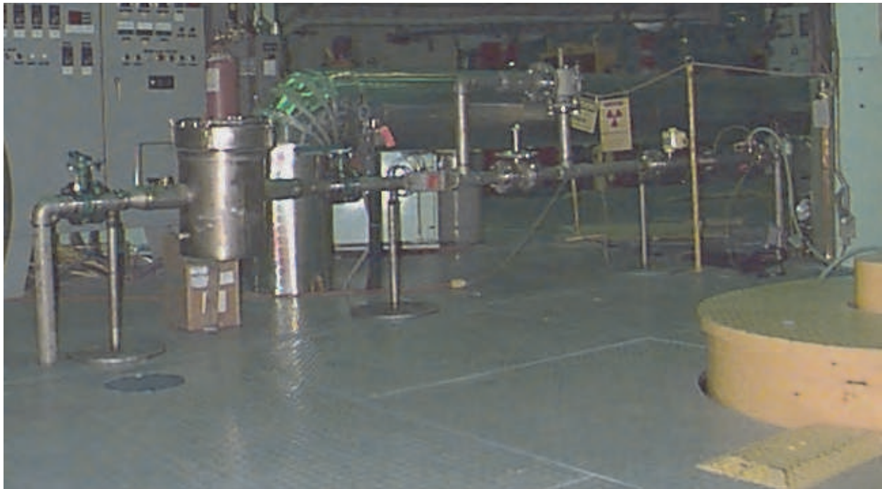
Fig. 8. Vent line for EBR-II Primary Tank with installed instrumentation and HEPA filter.
