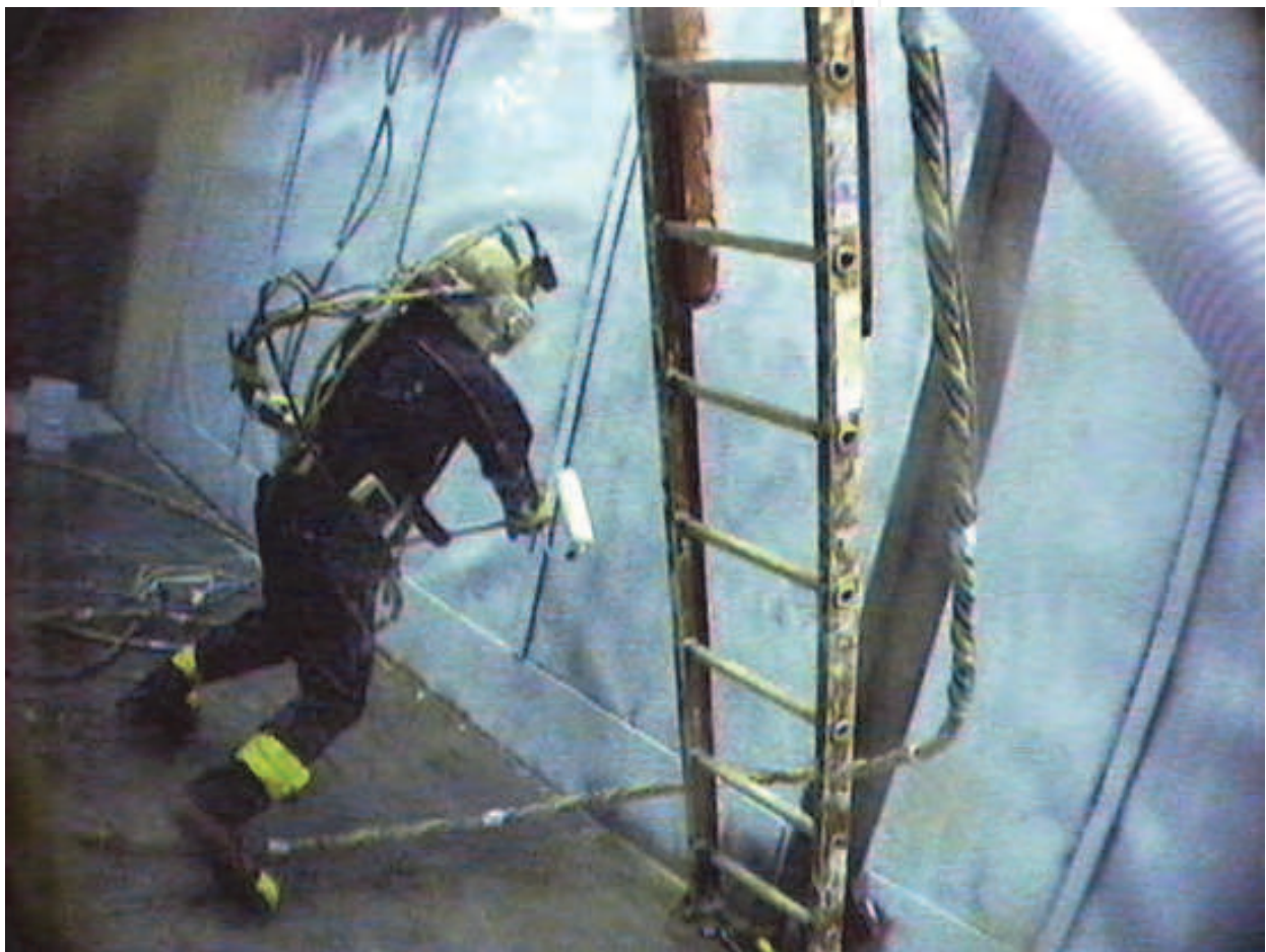
Fig. 2. Special two hose roller system used for wall coating at the MTR pool.
