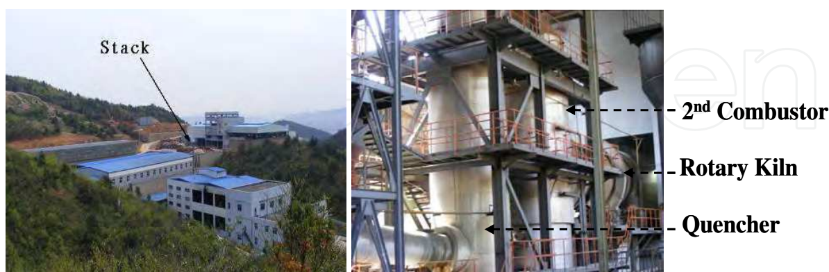
Fig. 1. Outside view and internal view of the medical waste incinerators.
