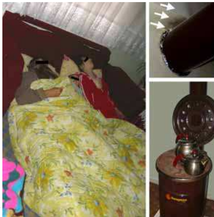
Fig. 23. A family (father, mother and child) was found dead in their bed due to carbon monoxide poisoning. There was a coal stove in the room and soot traces (arrows) were observed at the entry point of the stovepipe on the wall which indicating leakage of smoke of the stove.
