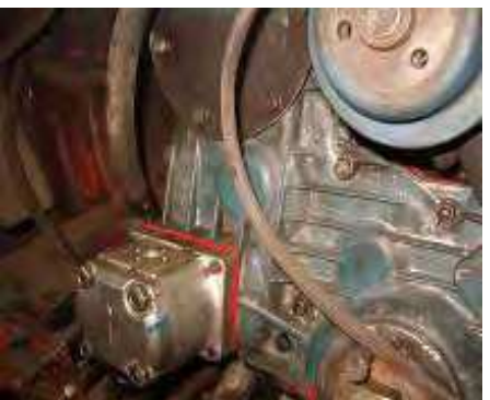
(f) Installation of the pump command
