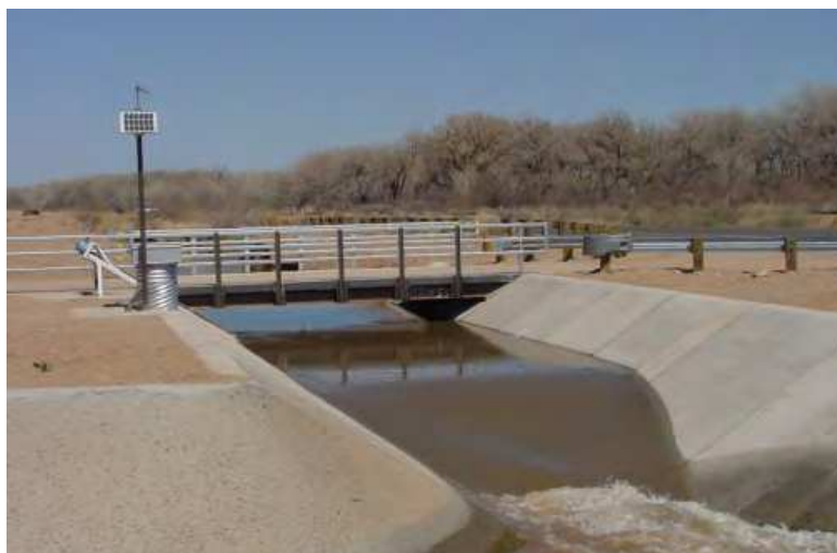
Fig. 10. Broad Crested Weir Gauging Station with Radio Telemetry
