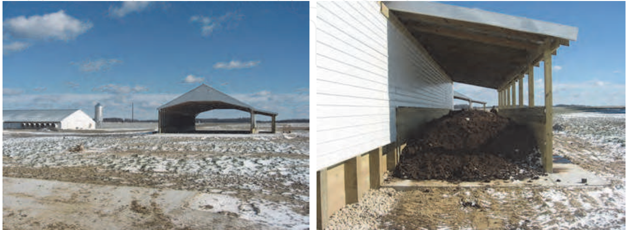
Fig. 3. Composting facility constructed on the side of manure sheds at poultry facilities, Delmarva Peninsula, USA. Photos: K. Wilkinson.
