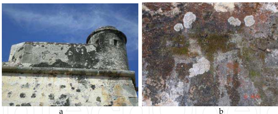
Fig. 11. Aspect of the biodeterioration in the historic buildings of San Francisco de Campeche City. (a) Fort San Carlos. (b). Microbial community at West wall of Fort San Pedro.
