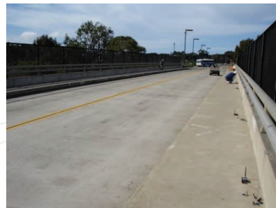
(c) Side view of the bridge over Interstate 5
