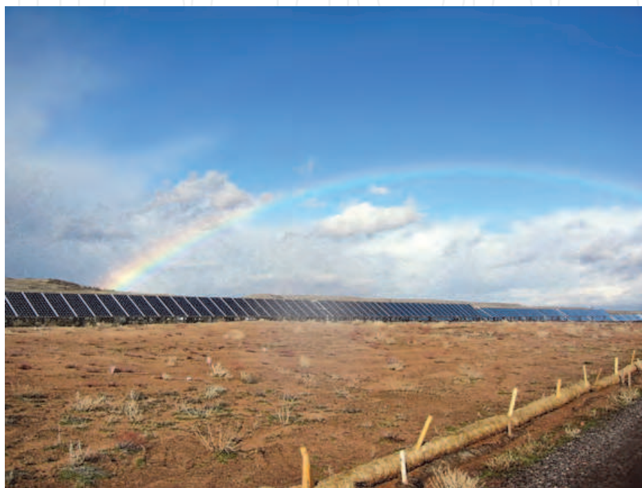
Fig. 3. PV system power plant of Tucson Arizona Public Service (photo by author)
