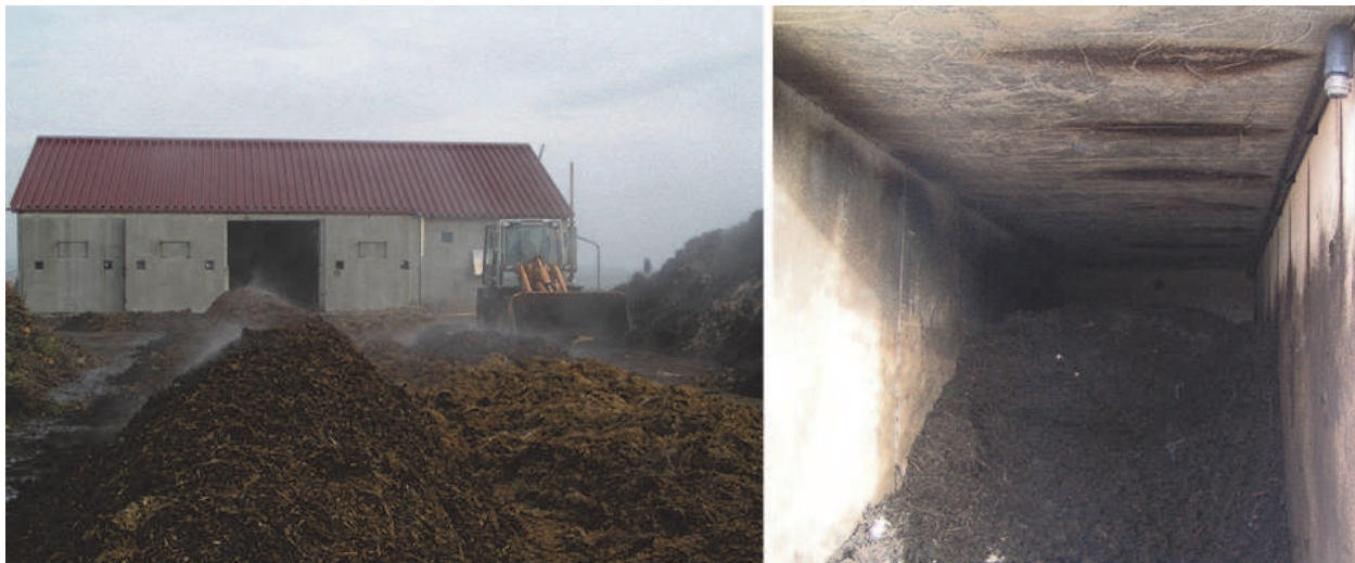
Fig. 3. Full-scale farm plant with four solid-phase digestion boxes
