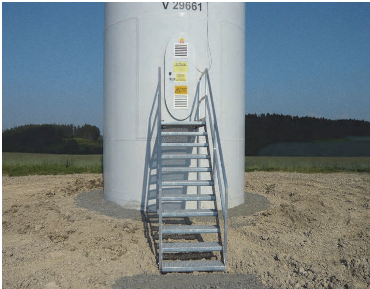
Fig. 5. View of the anchorage of the wind turbine pole into the anchor plate (Lapčík, 2008)
