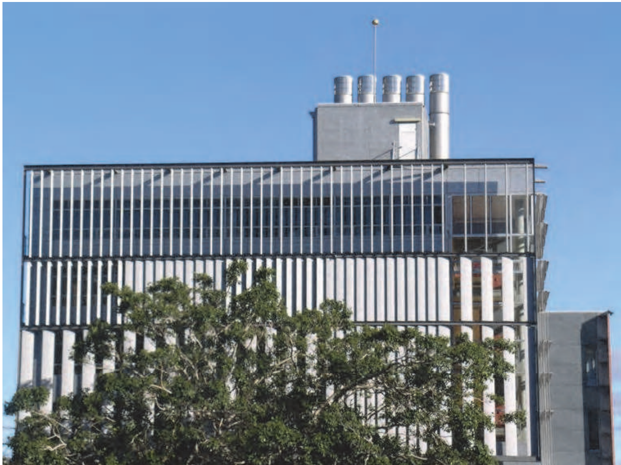
Fig. 16. Rotating ventilators in use on the roof top of building at the University of New South Wales
