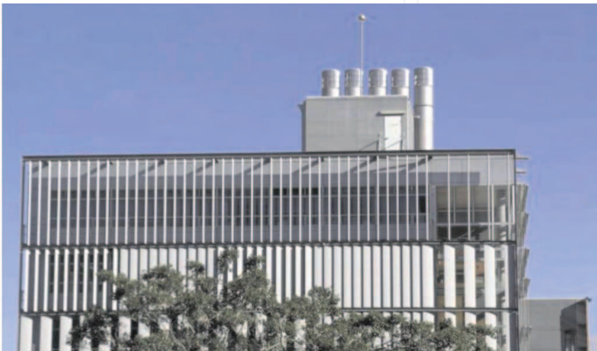
Fig. 2.5. Installation of multiple stacked ventilators at UNSW
