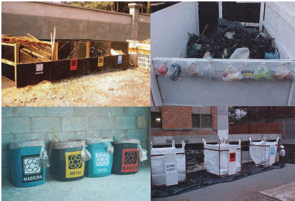
Fig. 4. Segregation of waste at the construction site
