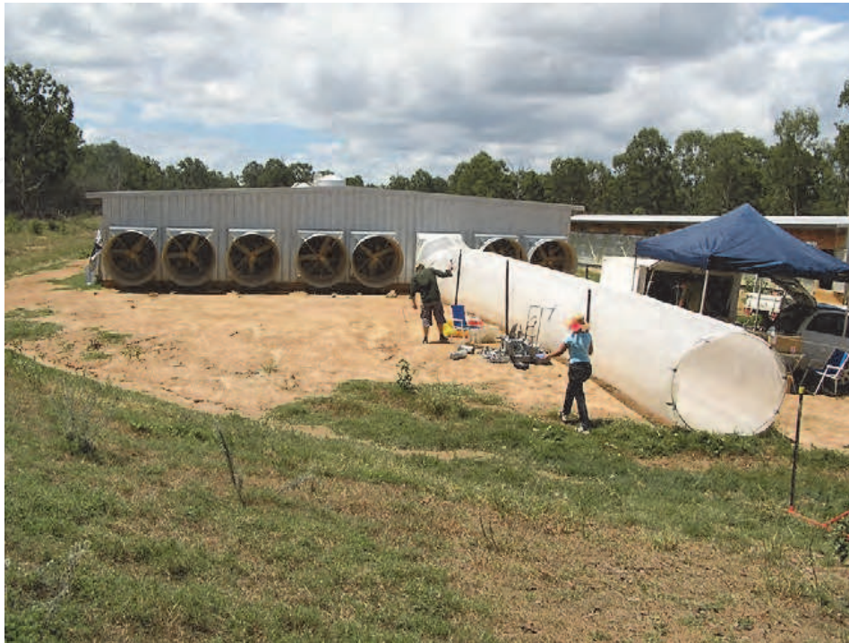
Fig. 4. Tunnel ventilated broiler shed showing polyethylene sampling duct attached to an exhaust fan. (Sohn et al., 2008)
