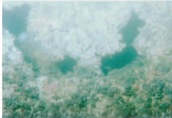
Fig. 1. An sample underwater photo taken during a pier inspection.
