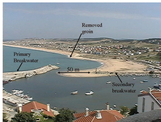
Photo 1. Karaburun Fishery Harbor and the nearby beach at east of Harbor (looking towards south east direction) (Ari et al., 2007)
