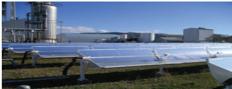
Fig. 23. ACUREX solar plant
