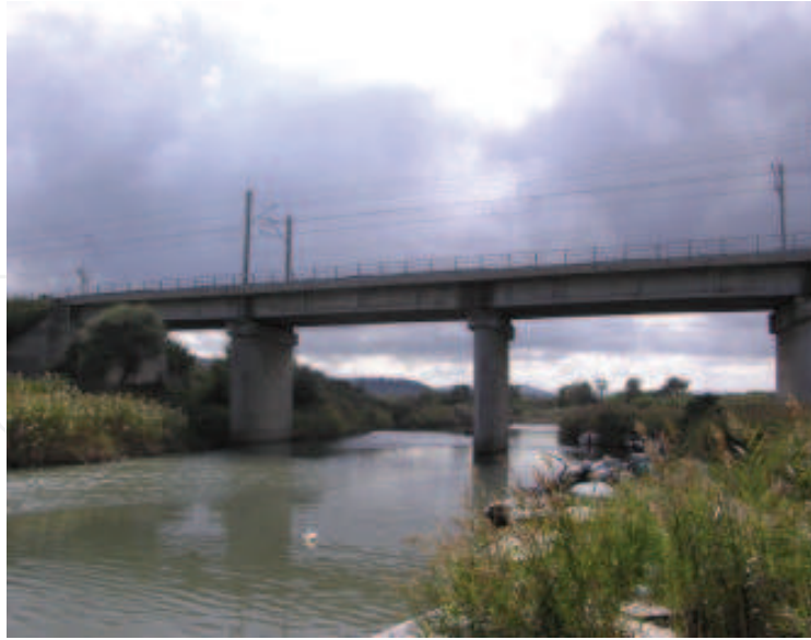
Fig. 1. Sinello railway bridge (Garibaldi et al., 2005).
