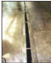
Photo 1. Dirty water generation: wash down high volume low pressure hose and drainage channel for speeding up washing after milking (Source: www.teagasc.ie )
