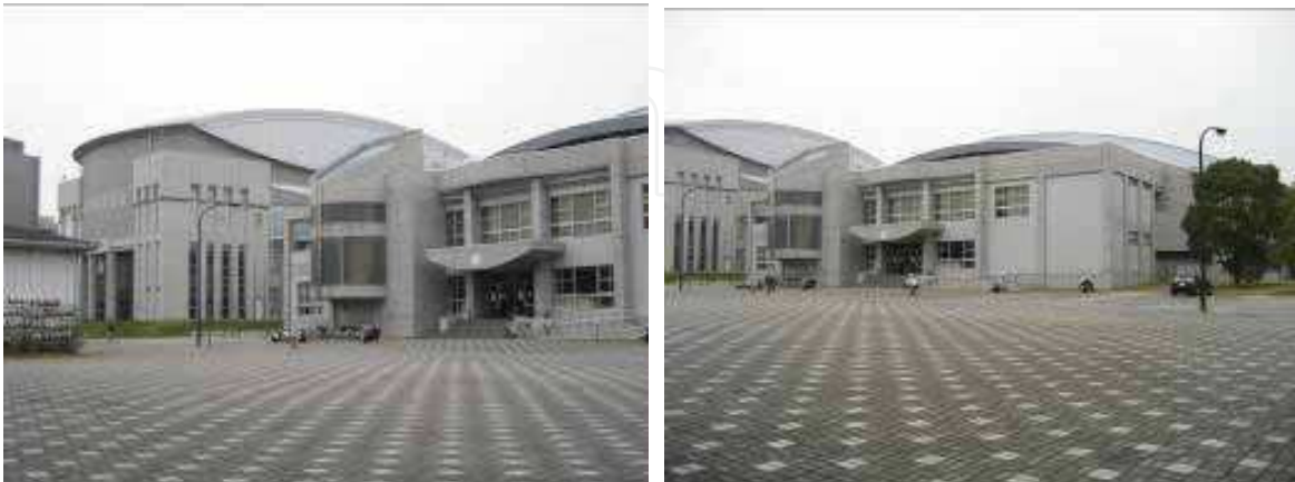
Fig. 6. Convention Center (left) and Gymnastic Hall (right) of Osaka University
