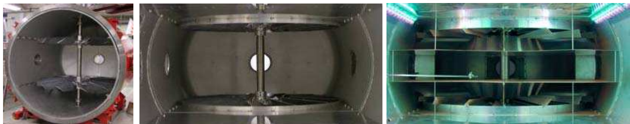
Fig. 6. Photographs into the flow generation section at the AWTS-II facility, Left shows the 1.8m diameter fans installed, Center shows with the upper and lower flow separators and Right the system of vertical and horizontal flow guides compartmentalizing the flow, preventing rotation and excessive turbulence.
