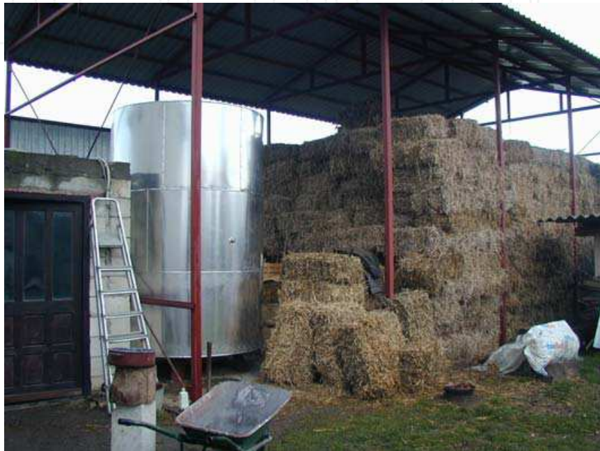
Fig. 6. Heat accumulator (thermal reservoir)
