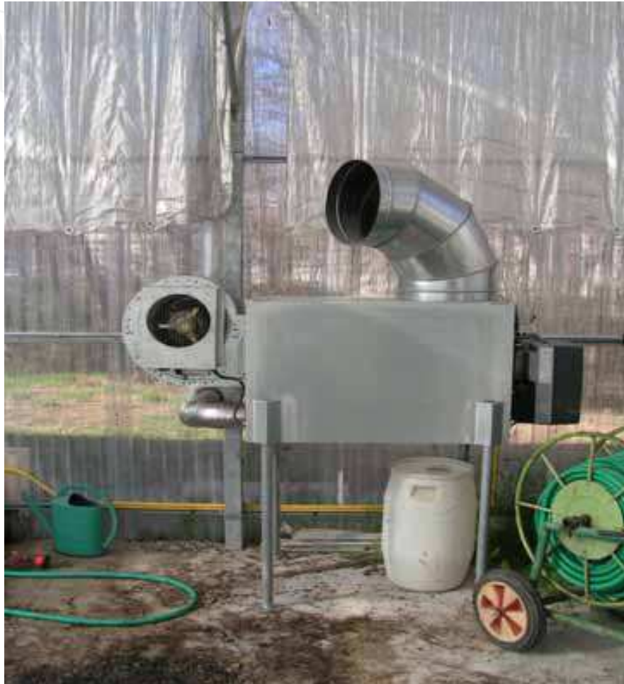
Fig. 3. A 55kW gas heater: extremely effective, but the gas is expensive and polluting
