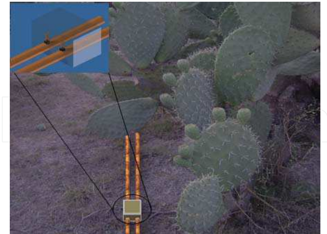
Fig. 16. Conductor in the soil and box connection
