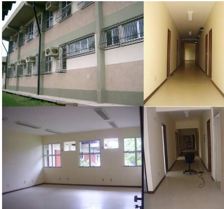
Fig. 2. Photograph of the research laboratories building: corridors of the second and first floor, and laboratory classroom
