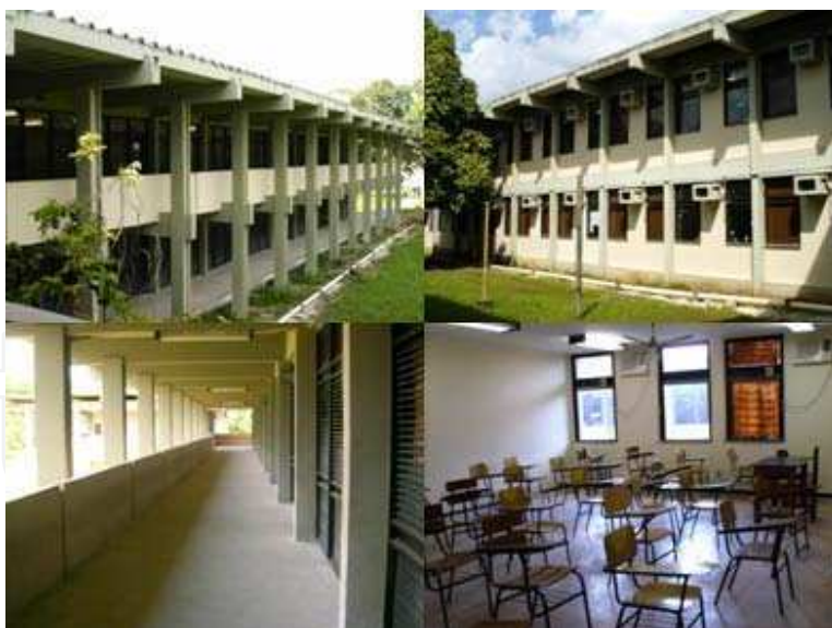
Fig. 1. Photograph of the building. In clockwise: external side with glass windows, classroom, corridor and external side with corridor along
