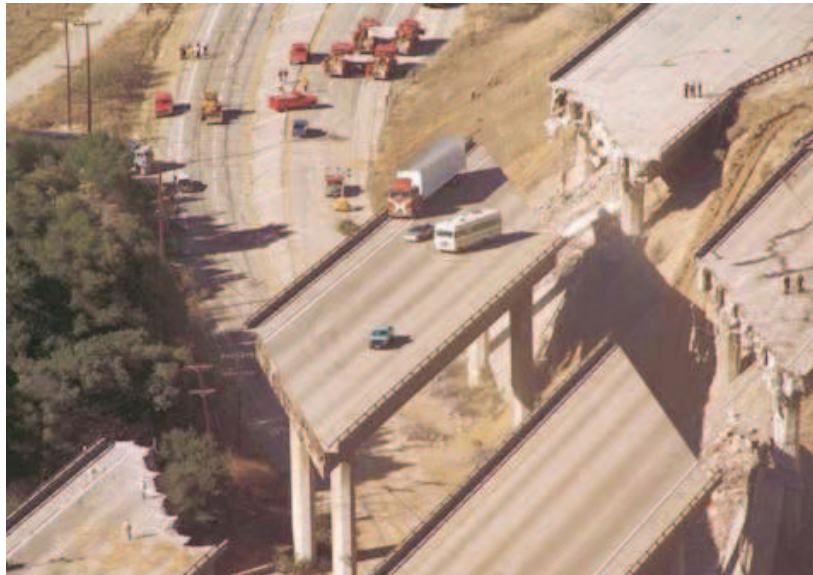
Fig. 3. Example of bridge collapse after an earthquake
