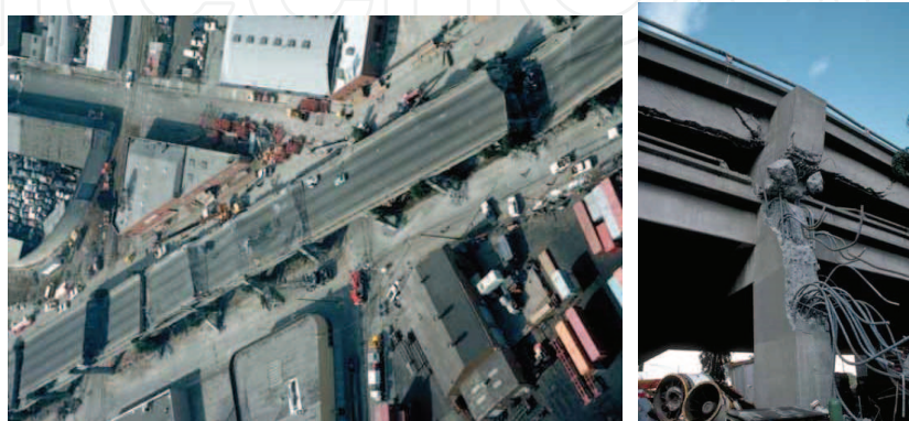
Fig. 1. Loma Prieta, sections of the Cypress viaduct (H.G. Wilshire, U.S. Geological Survey)
