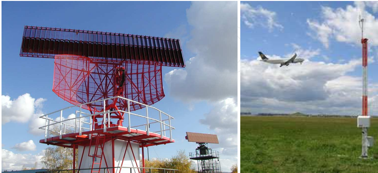
Fig. 1. Primary and secondary surveillance radar (picture source: author)
