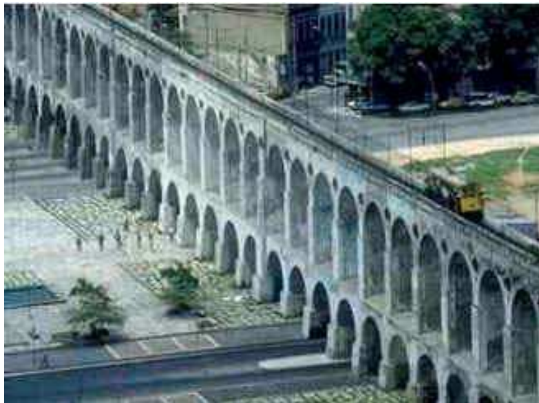
Fig. 1. Arches of Lapa, aqueduct where Carioca River ran in the past
