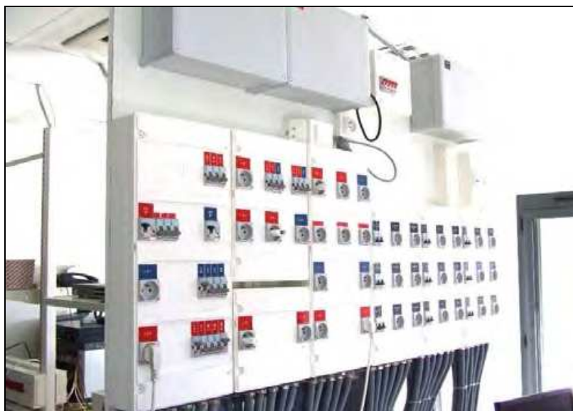
Fig. 2. PLC test environment available in DAL
