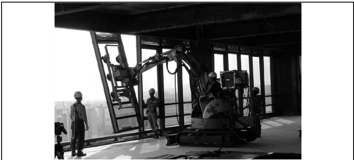
Fig. 2. An ASCI (Automation System for Curtain-wall Installation)
