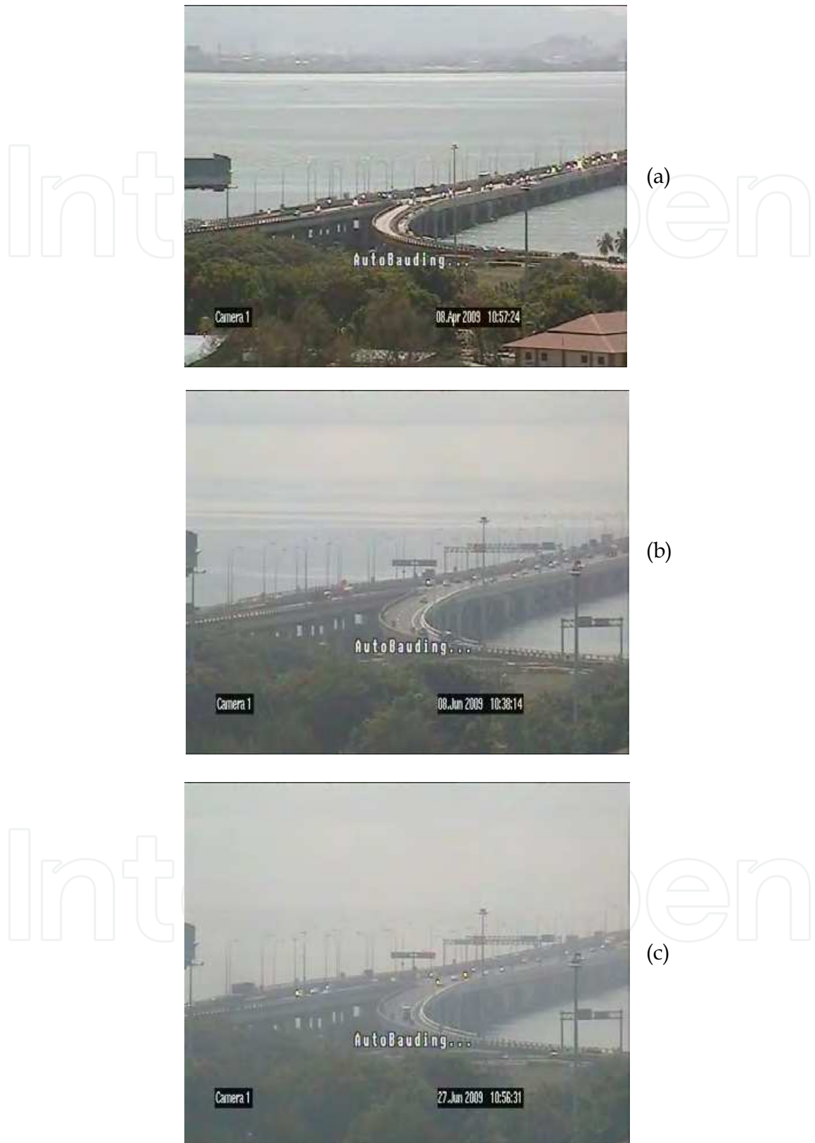
Fig. 7. Three photographs of Penang Bridge at different atmospheric aerosol concentration level
